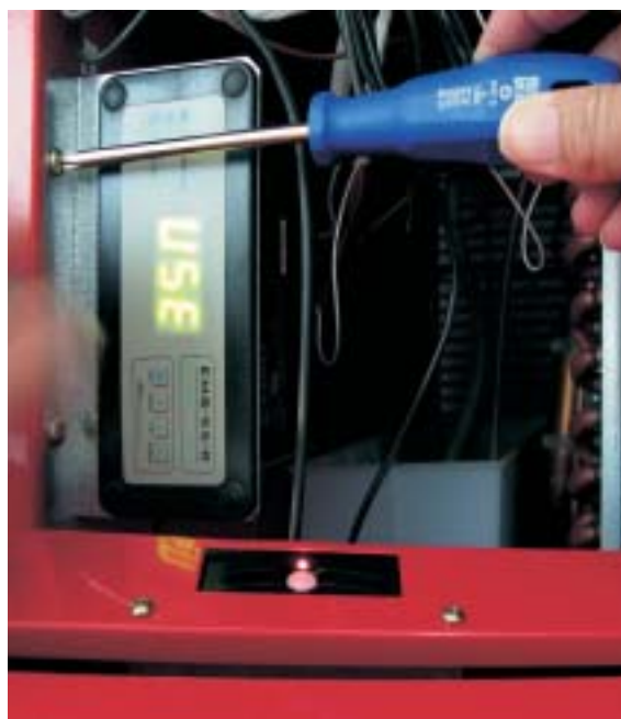
Energy saving devices for cooling equipment like this EMS-55 unit record events such as passing consumer traffic, door opening frequency and store downtime then adjust compressor and light usage accordingly began being installed in refrigeration equipment from 1 January 2007.
